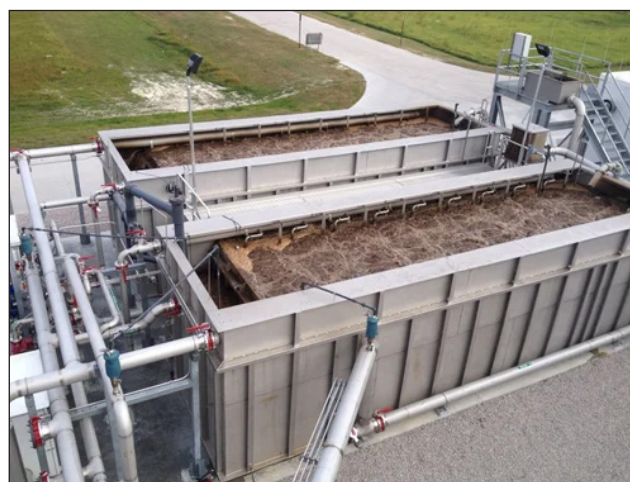
Figure 4: Membrane bioreactors used in wastewater treatment
